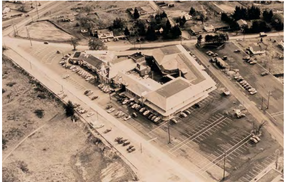
Lakewood was still more prairie than populated when this picture of the recently completed Colonial Center was taken in 1951.
